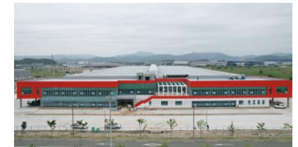
산업설비 (Industrial Facility)
