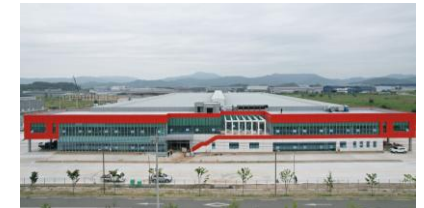
산업설비 (Industrial Facility)
