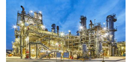
화학 (Chemical Plant)
