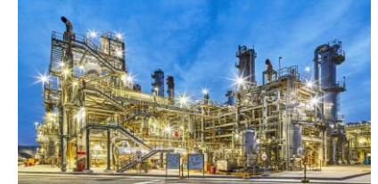
화공 (Chemical Plant)
