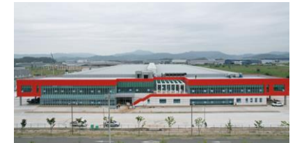
산업설비 (Industrial Facility)
