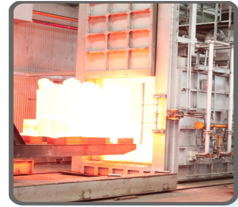
HEAT TREATMENT FURNACE
